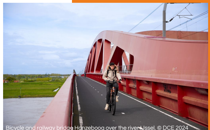
Bicycle and railway bridge Hanzeboog over the river IJssel. © DCE 2024
